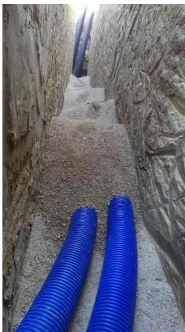
Air tubes with diameter 20cm
