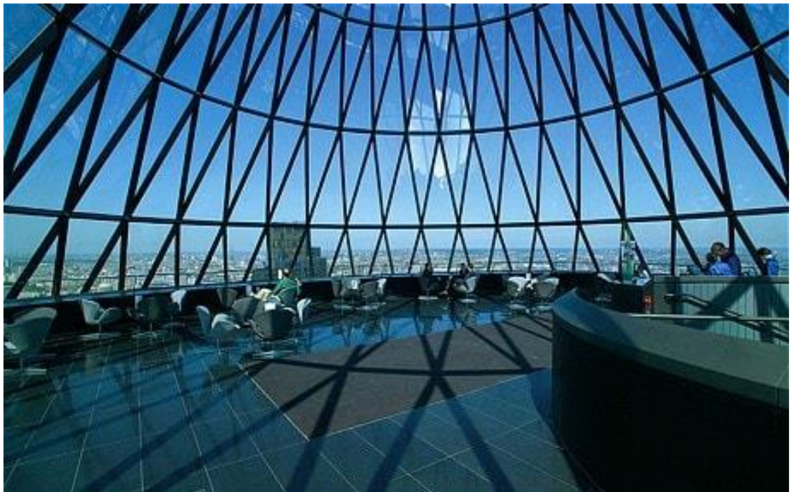
The building is designed by Roman Foster. Every floor is shifted 5 degrees from the one below
